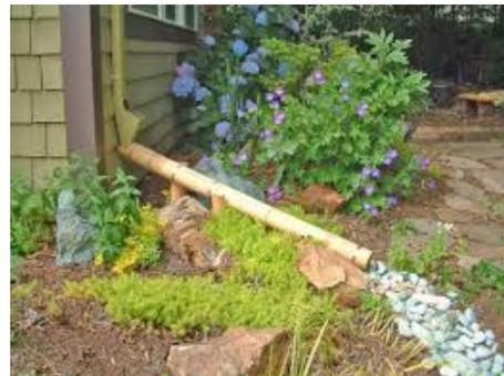
**Figure 13. Downspout Disconnection**
