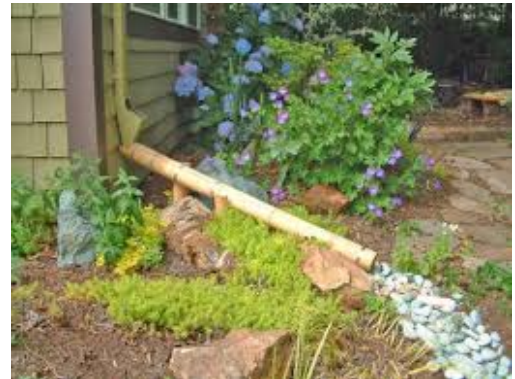
Figure 13. Downspout Disconnection
