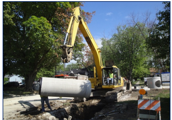
Figure 15. Typical Storm Sewer
